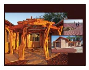
Architect Daniel Glenn and colleagues at Arizona State University built a model sustainable home in Nageezi, New Mexico. The model home incorporates design elements of the traditional Navajo *hooghan*, such as passive solar temperature control and thick walls for added insulation from the desert heat. The corbelled cedar pergola over the central courtyard mirrors the distinctive architecture of the *hooghan*.
