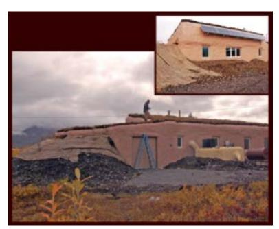
Designed to withstand harsh weather conditions on Alaska's North Slope, the Anaktuvuk Pass Prototype Home is modeled on traditional sod igloos of the region and features an earthen roof, spray-foam-insulated exterior walls bermed into the earth, a passive ventilation system called a *qingok*, and solar panels to supplement grid electricity. An unheated cold room stores game, a staple of the local diet.
